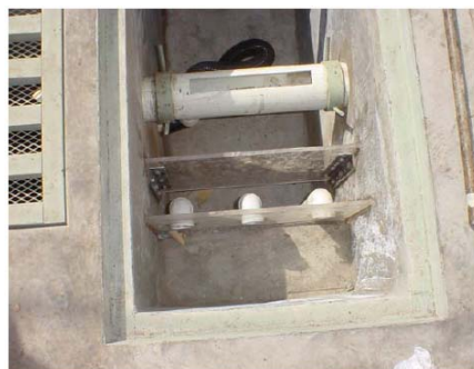
Fig. 2: Photograph that shows the details of the skimmer, oil baffle and outlet weir of the Prototype separator
